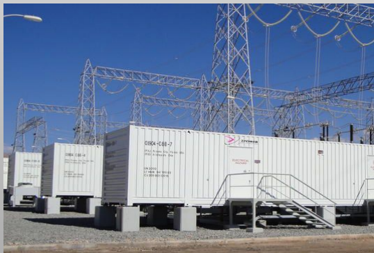
Utility Substation Installation
